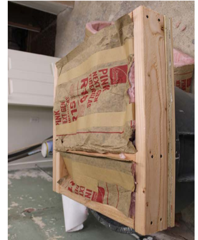
Appendix C3 Figure 6 - Sample 3 construction showing framing and insulation.
