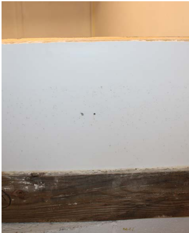
Appendix B3 Figure 11 - Sample 2 after the extended drying period.
