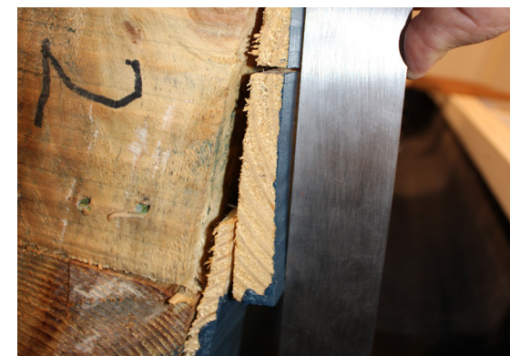
Wall Assembly 2 (Wire Lath & Plaster) showing split siding post-drying
